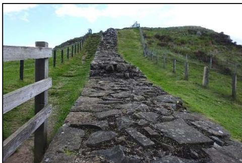
A preserved section of Hadrian's Wall near the museum. Roughly 10% of the original wall is left. Average height was 15' and width started at 9.5', but was reduced to 7.5' as construction progressed.
